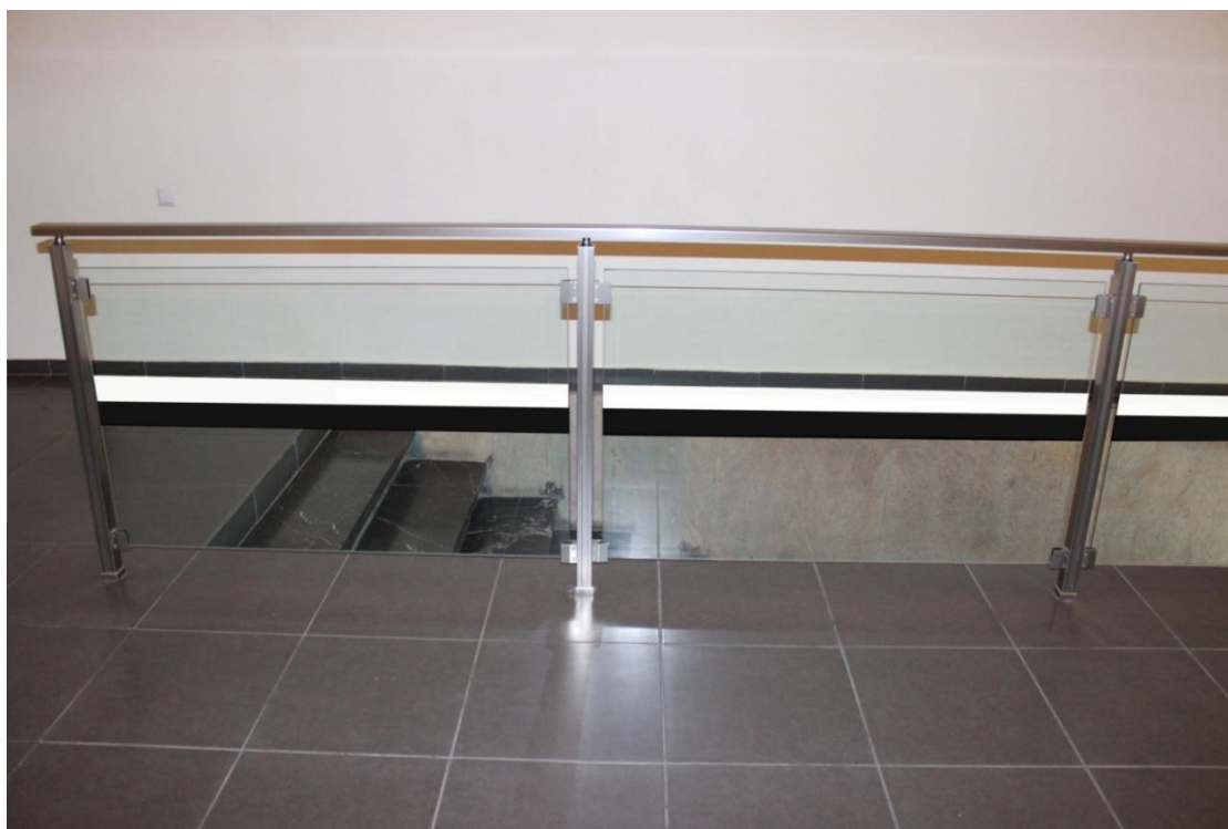
Photo N 14: Glass handrail at the cinema hall staircase – innovated - project
